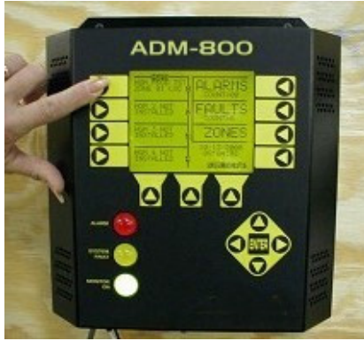
Figure 5. Push button of monitor being serviced to display its SETUP Screen
